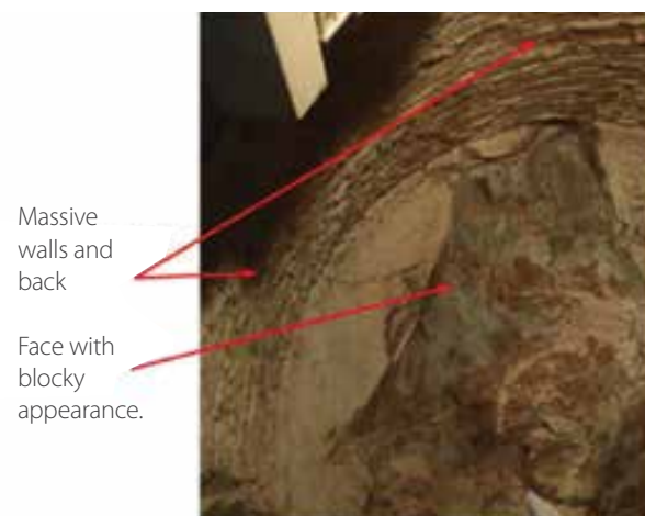
Figure 1. Blocky appearance of rock in TBS tunnel face at Northparkes Mine resulting from veined nature of rock.
