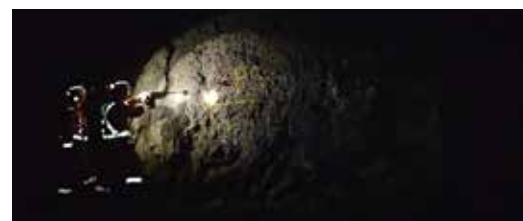
Drilling preparation for the installation of seismic sensors at Nickel Rim South Mine with Christopher Carlson & Ko Korenromp
